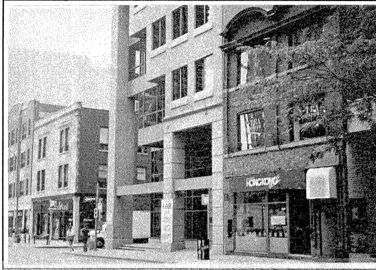
Ste-Catherine St., south side: a mix of old and new buildings of high density.
